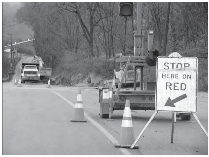
Work begins on laying the pipe at Carl.
