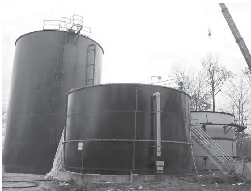
The tallest tank is the Clearwater tank; the two others are the pre-sediment tanks.
