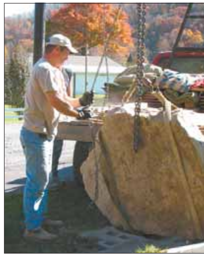
Wes Sheridan at work installing a new sign at Pratt Park.
