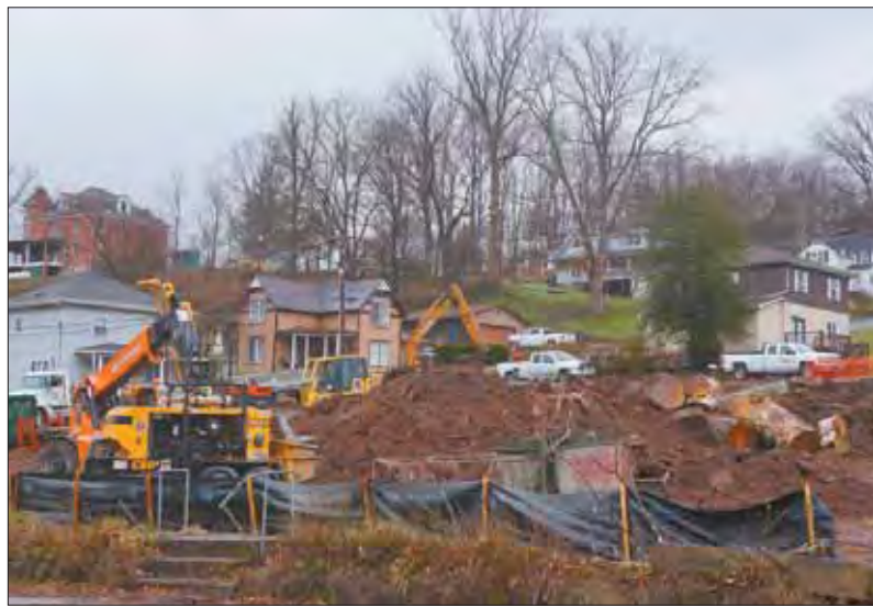
Construction is well underway at the site of the new Dollar General Store in Webster Springs.
